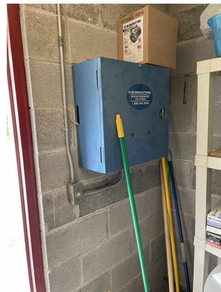
EXHAUST FAN CONTROLS SEE NOTE 1
