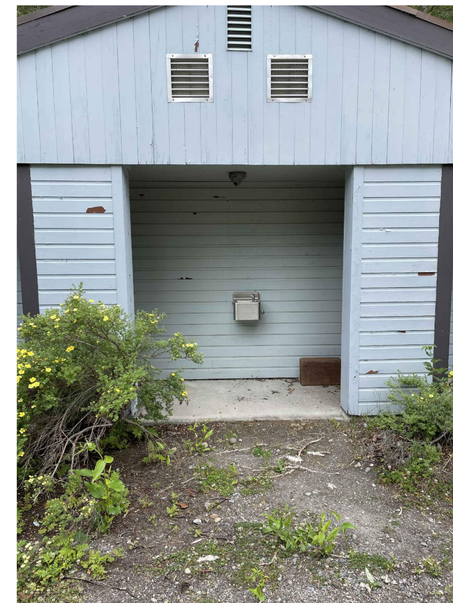
WEST SIDE BUILDING WITH DRINKING FOUNTAIN
