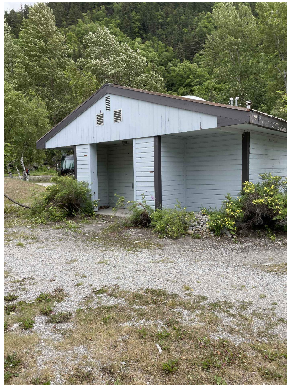
WEST SIDE BUILDING
