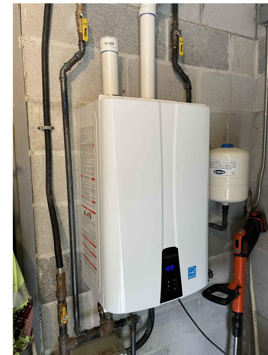
SALVAGE GAS HOT WATER HEATER SEE NOTE 1
