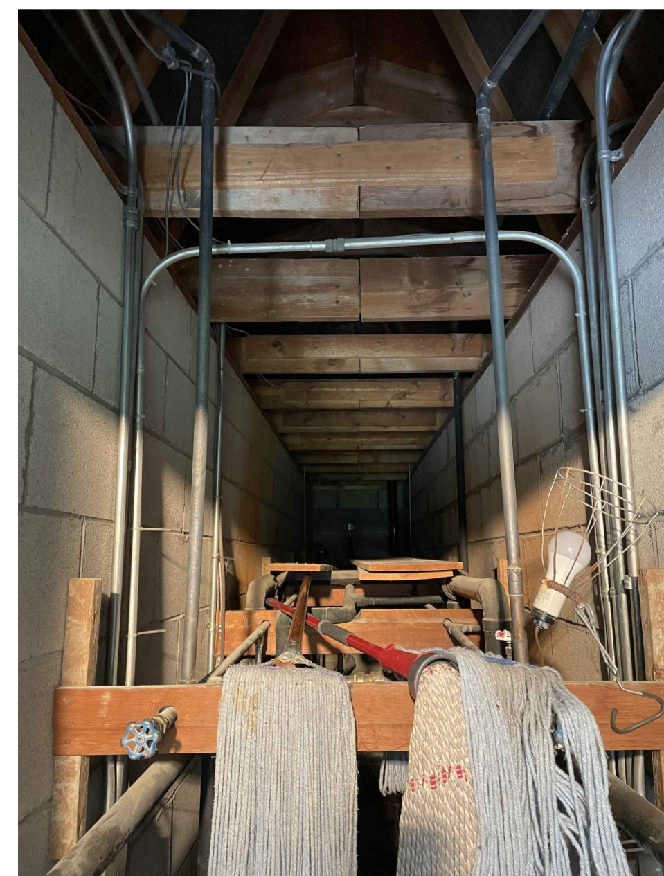
MECHANICAL CHASE WITH WOODEN TRUSSES ABOVE CMU WALL
