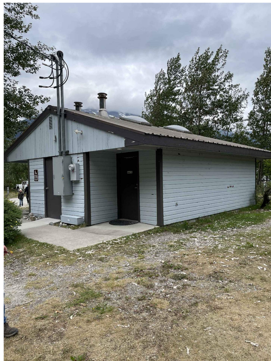
EAST SIDE BUILDING ENTRANCE
