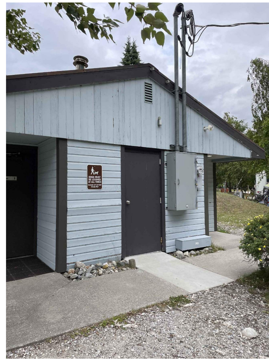
EAST SIDE BUILDING ENTRANCE
