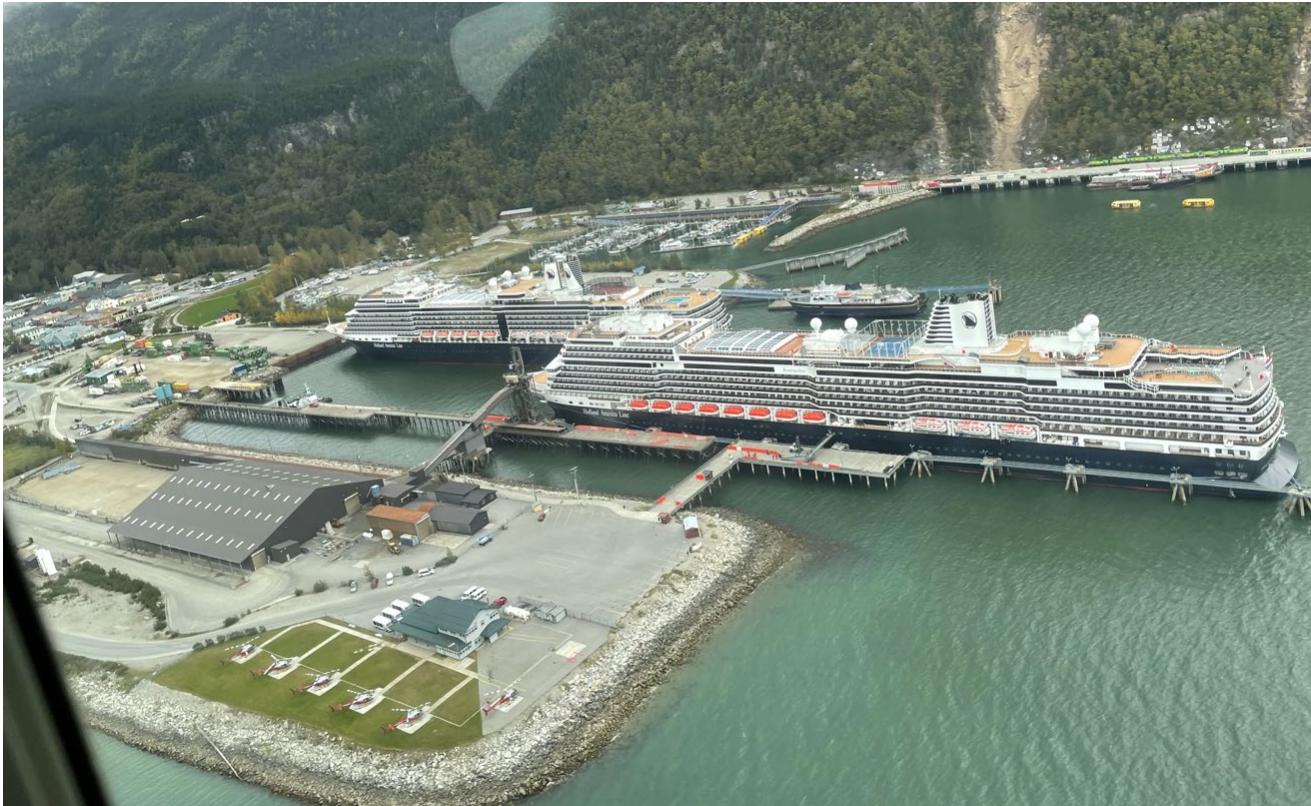
Figure 2.4 Skagway Waterfront showing subject upper photo left of slide. Photo 9/20/2022.
