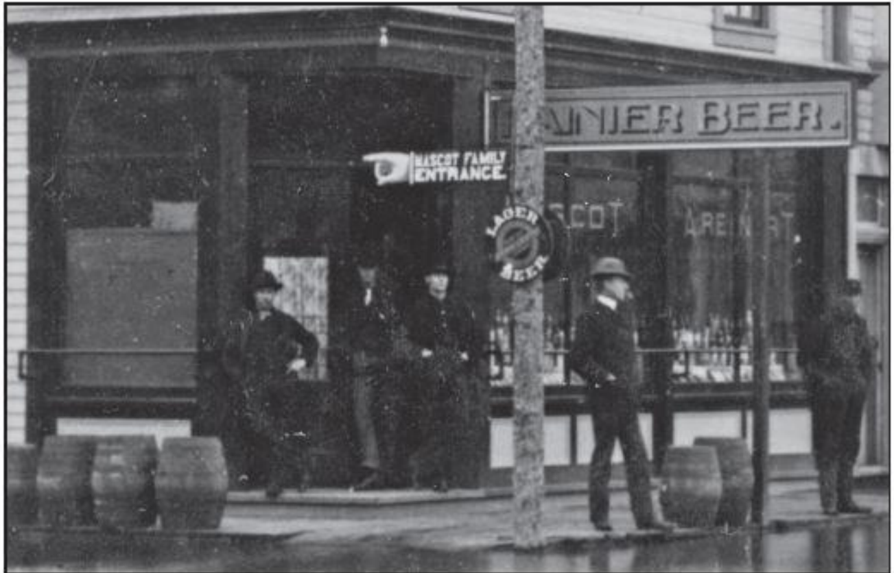
Figure 24b: Detail, Mascot Saloon front entrance, looking southeast. Date: 28 October 1901.
