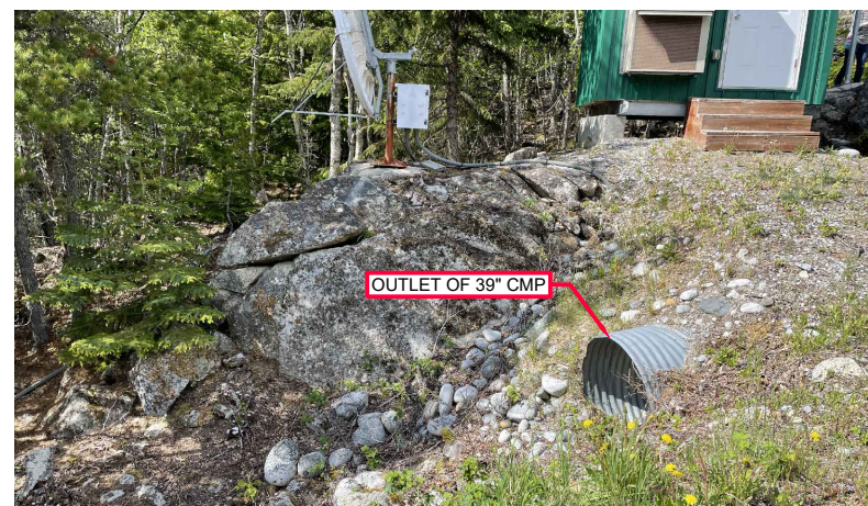
4 OUTLET OF 39" CMP CULVERT - VIEW LOOKING WEST
