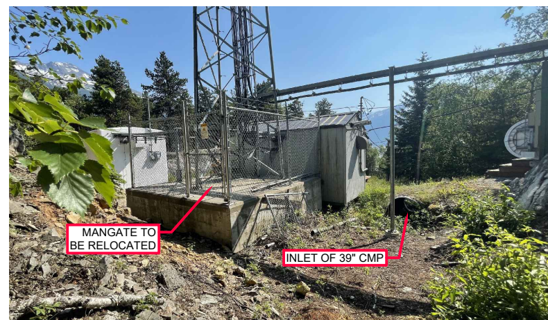
7 FENCE AROUND AT&T TOWER - VIEW LOOKING SOUTH
