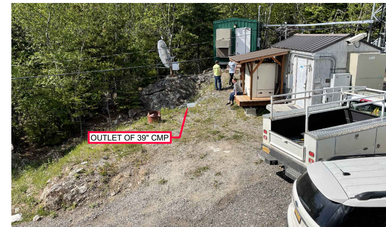
3 GCI AND AT&T BUILDING - VIEW LOOKING WEST
