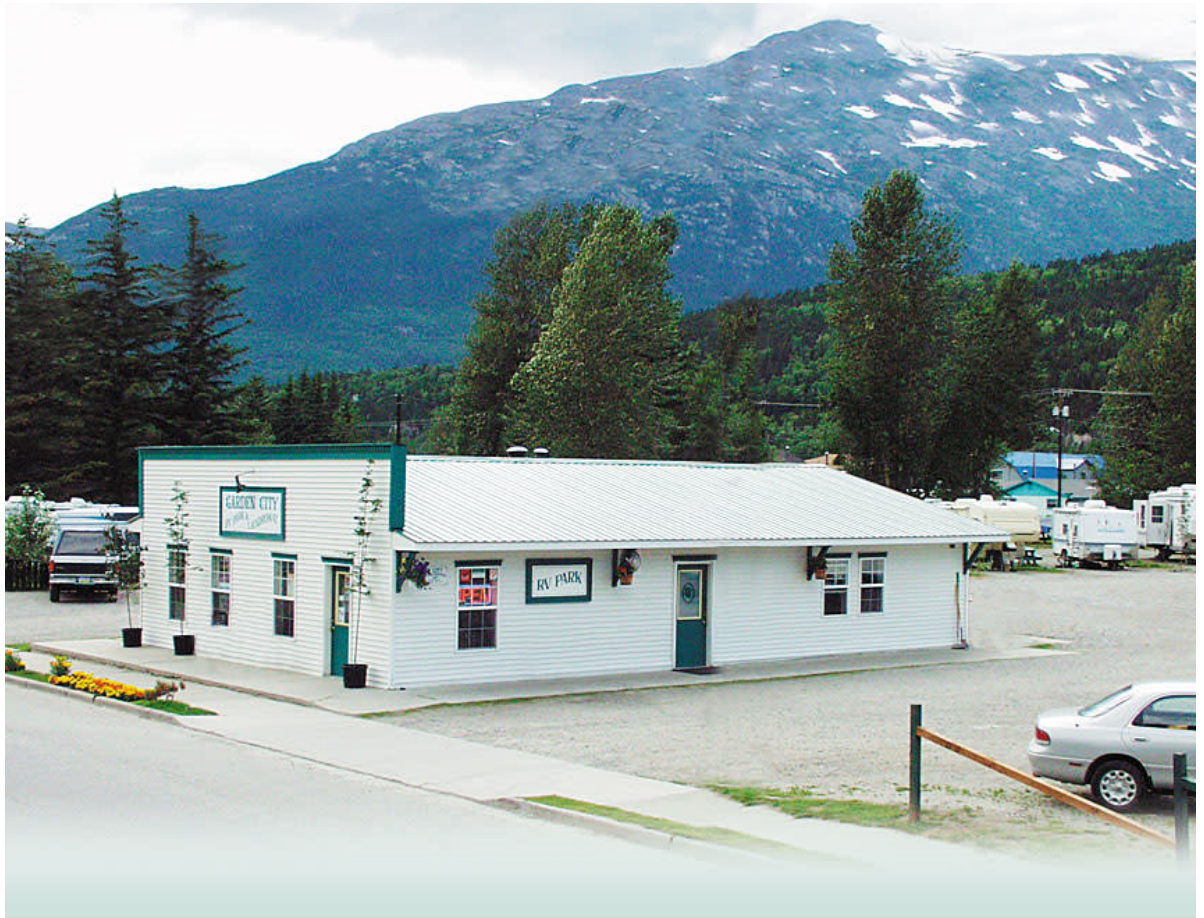
Garden City R/V Park Laundromat and Restroom Building
